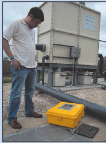
Bag sample collection at inlet duct
